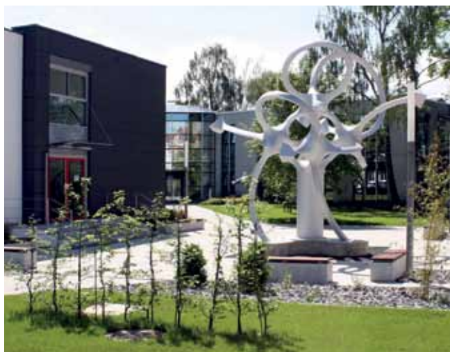
Fig. 1: Administration Building, Zwick Roell AG and Zwick GmbH & Co. KG, Ulm
